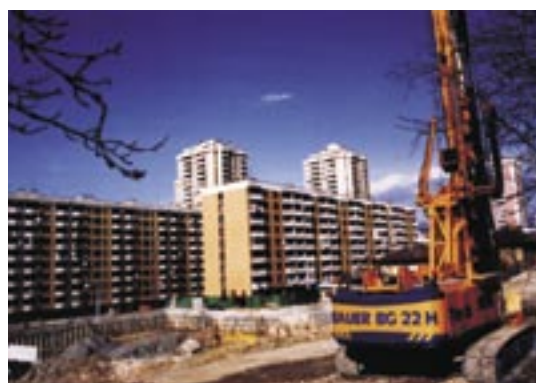
Residential housing under construction
